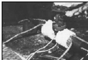
**FIGURE 3 Insulation of a 1/2" Valve Body for PWHT**
